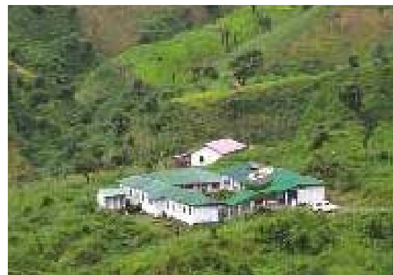
Primary Health Care Centre in a remote region of Arunachal Pradesh run by Karuna Trust
